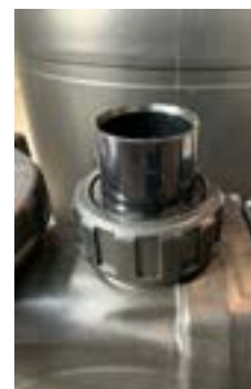
RACCORDEMENT POMPE Ø50
