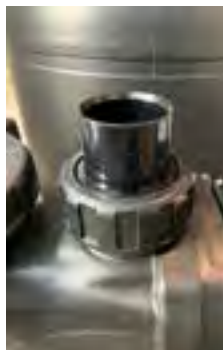
RACCORDEMENT POMPE Ø50
