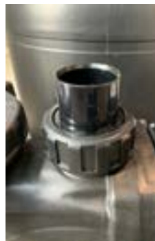
RACCORDEMENT POMPE Ø50
